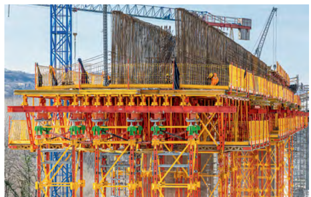
The PROKIT Guardrail provided site personnel with protection against open building edges at all times.
