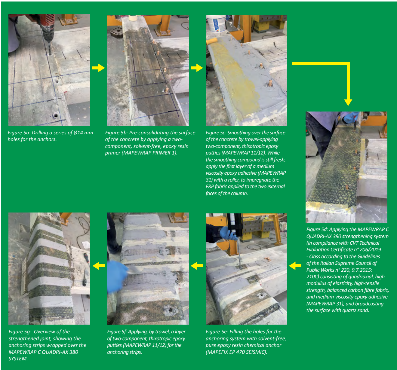
Figure 5: Steps in the application of the FRP strengthening system - external application only.
