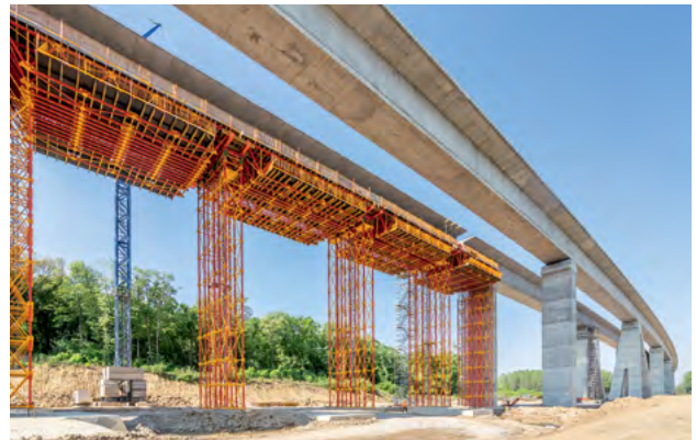
In Section B, the ALPHAKIT Shoring Construction Kit was chosen specifically because it is designed for a support height of up to 30 m.
