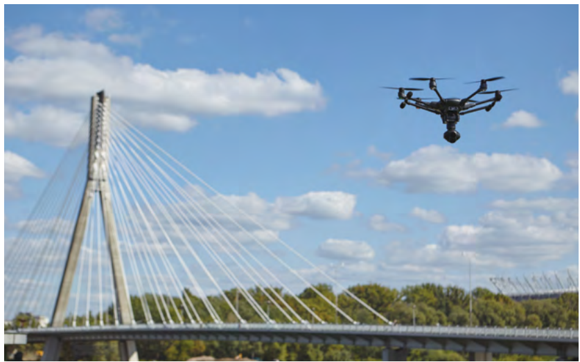
A drone inspects a bridge from above. Image: Bentley Systems.
