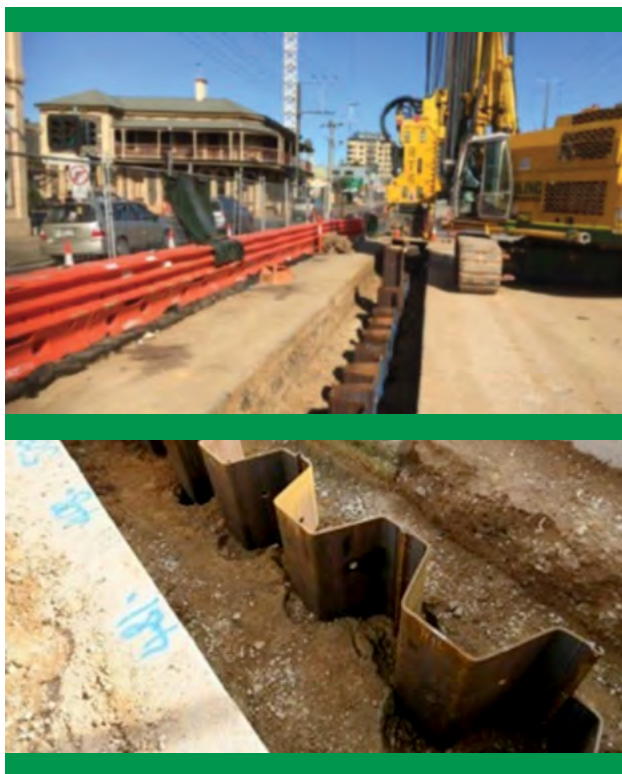
Picture 2: Application as a road retaining wall in Australia.
