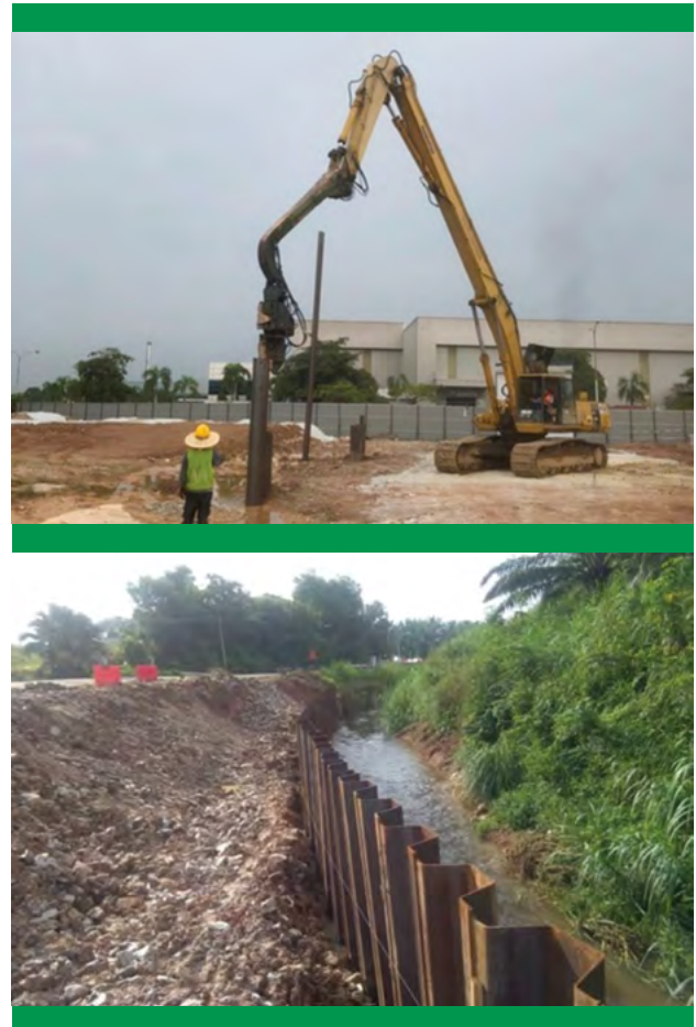
Picture 3: Application in Malaysia as temporary wall (top) and as river revetment (bottom).
