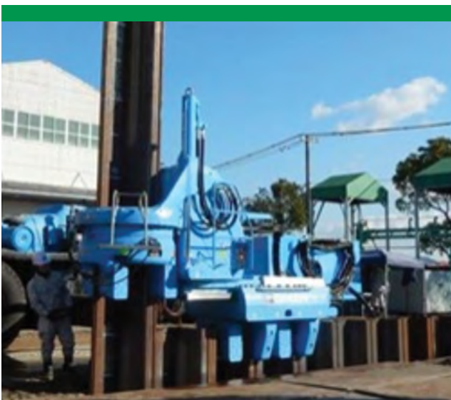
Picture 5: Silent piling in a city area (left) and in a residential area (right).
