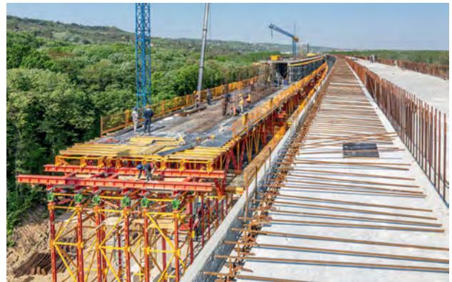
For concreting the two-lane superstructure, ALPHAKIT was supplemented in Section B with components of the MULTIFLEX Girder Slab formwork.
