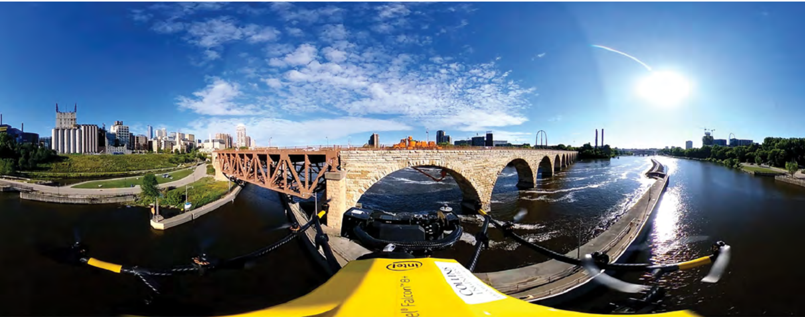
An unmanned aerial vehicle (UAV) acquires images of a stone bridge.
