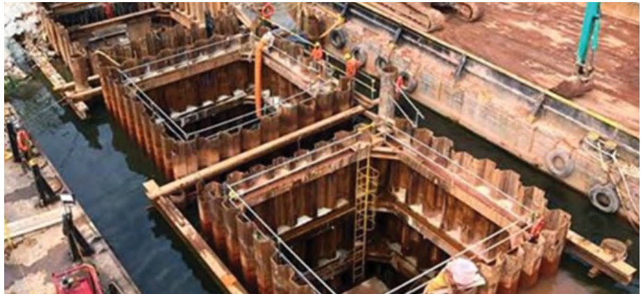
Picture 1: Track record for cofferdam on the seaside. Image: Steadfast Engineering & Construction Pte Ltd.
