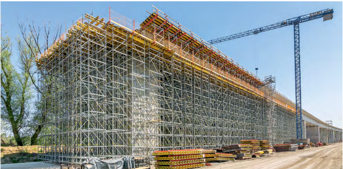
PERI UP supported the MULTIFLEX Girder Slab Formwork with a support height of up to 20 m.
