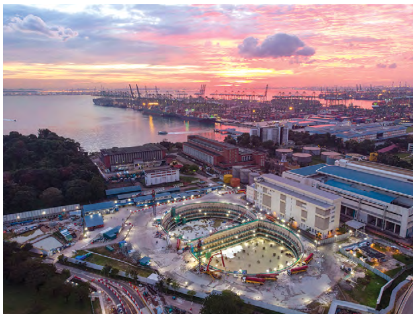
Pan-United delivered a total of 37,258 m 3 of concrete in two continuous mass pours.
